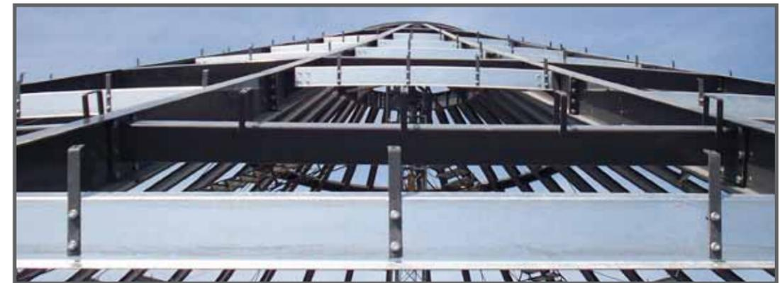
The roof panels are attached to the roof skeleton with standing seam roof straps (above) minimizing penetrations in the valley and creating a more weather tight roof. The roof panels are rigidized (right) across the entire width to produce a more rigid panel for longer life. The roof panels attach with numerous bolts to the wall system through a continuous angle (below) at the eave. This Behlen feature prevents roof panels from tearing loose in high wind conditions.
